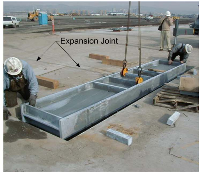
Beam Installation
