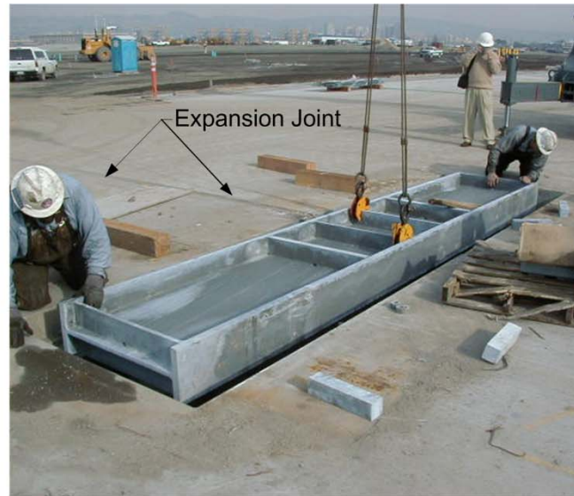
Beam Installation
