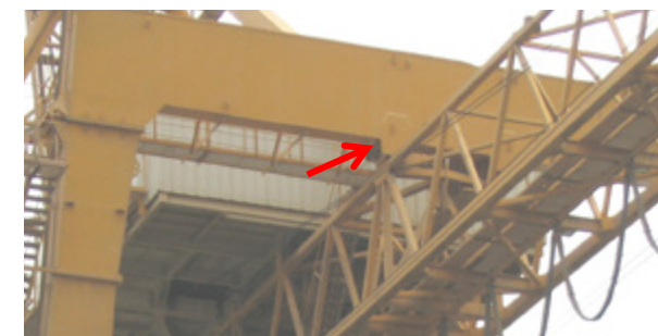
Picture 3.22: LS TGSB of a truss boom crane, in this case without radii at the points of transition.
