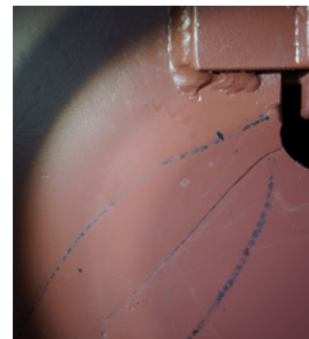
Picture 3.9: A crack in the inside diaphragm at a transition in the portal beam.
