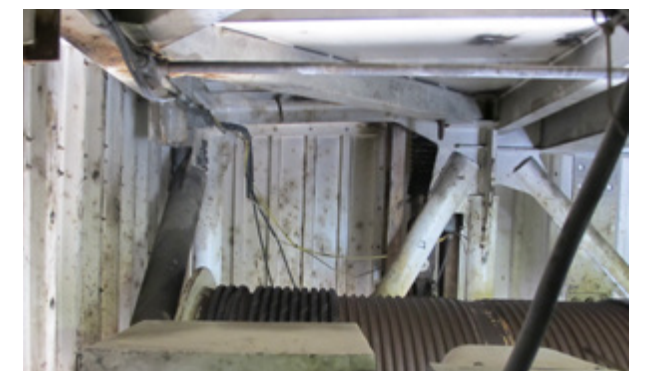
Picture 3.63: Trolley members inside machinery house.
