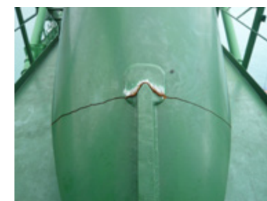
Picture 2.1: Crack in FCM at lower end of single upper diagonal pipe.
