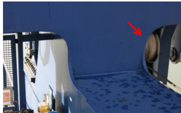
Picture 3.17: Welded TGSB to girder connection on twin girder crane with curved transition details to minimize stress concentration.
