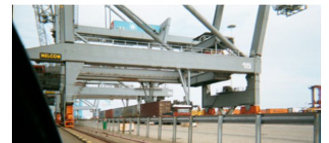
Picture 3.12: Sill beam, lower legs, and portal beam. Note landside lower legs are pinned at the portal. In this case, all horizontal loads are taken by the waterside legs, on the left.
