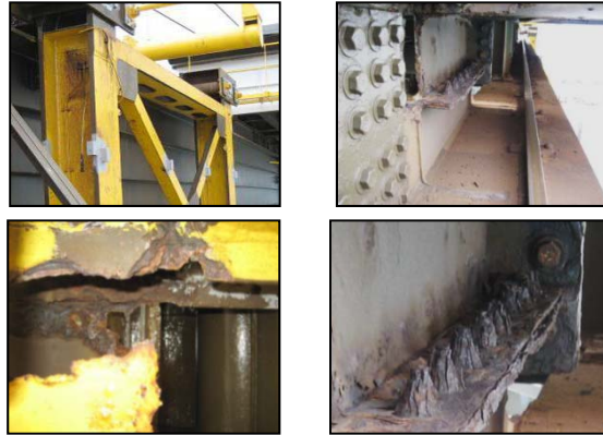
Corrosion Damage
