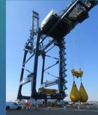
Load Testing, Pile Testing
