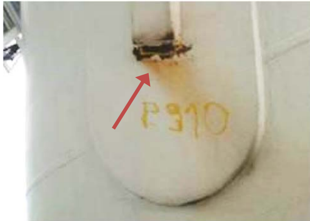
Figure 6: Cracking at the weld of the seal plate
