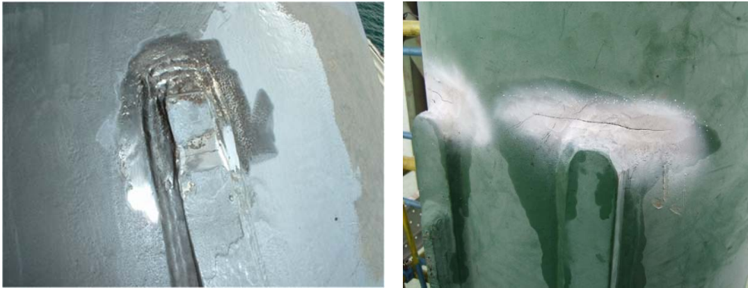
Figure 3: End connections with no stress relief hole, square cut without reinforcing plate (left) and with seal plate and fatigue cracks (right)
