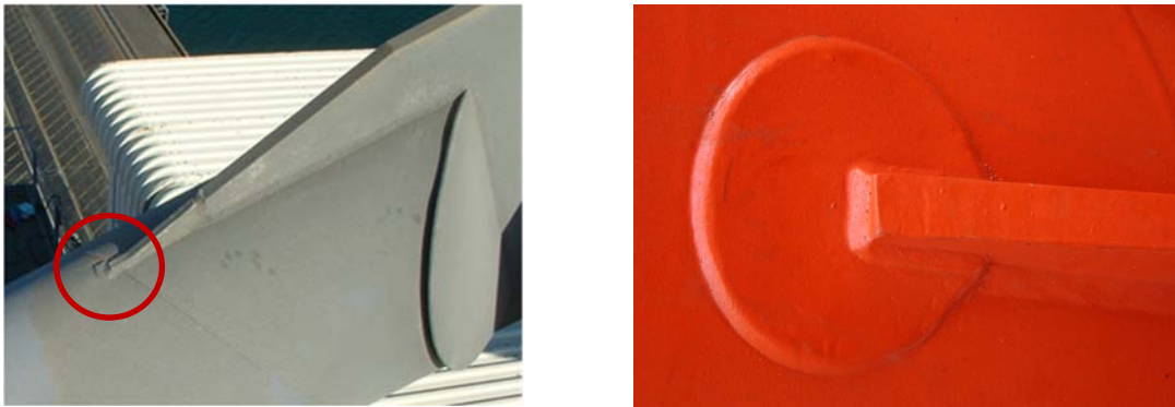
Figure 1: Pipe-to-gusset plate connection, without seal plate (left) and with seal plate (right)
