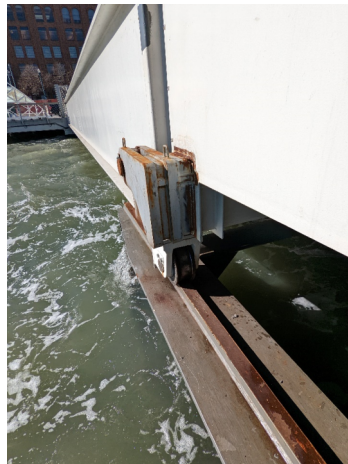
Roller supports at access ramp to float
