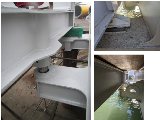
Kingpin and sliding supports at pier to access ramp
