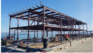
Building fabricated on float at Treasure Island
