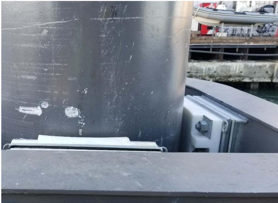
**Figure 10. Pile collar damper.**
