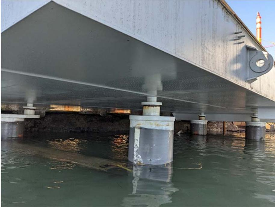
**Figure 2. Pier connection to pier piles.**
