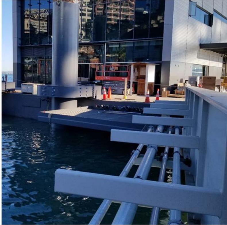
**Figure 6. Utility supports on access ramp and float.**
