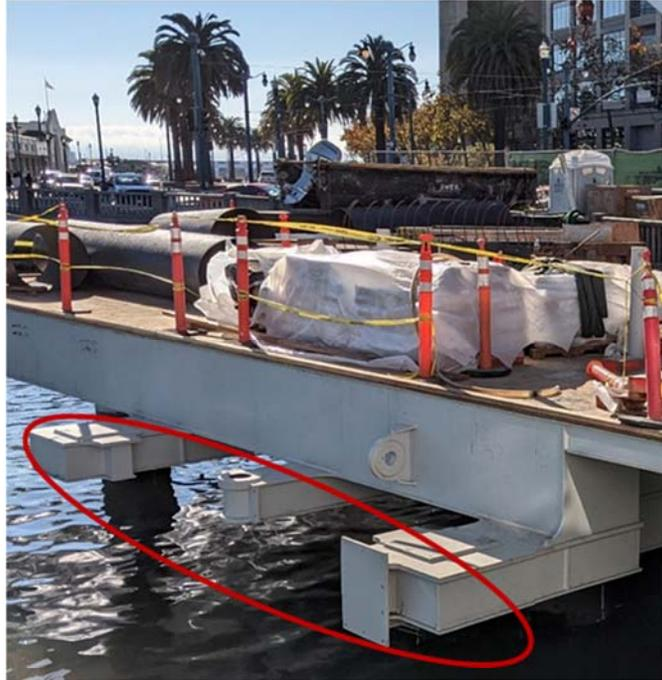
**Figure 7. Pier kingpin sleeve and slide bearing supports.**
