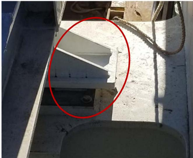
**Figure 8. Interface of access ramp sliding foot and pier (Teflon bearing).**
