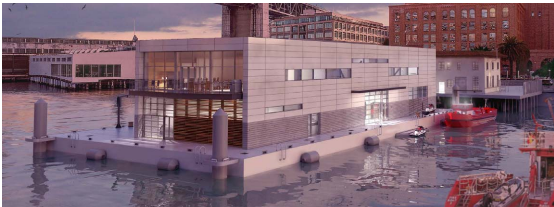
Figure 3. Steel float with building on deck—System 3
