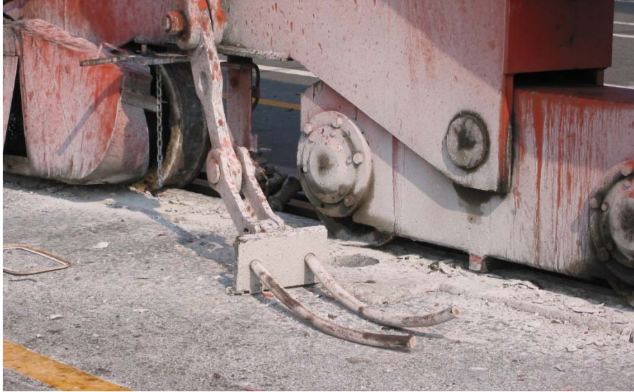
Figure 4. Wharf Anchorage Failure
