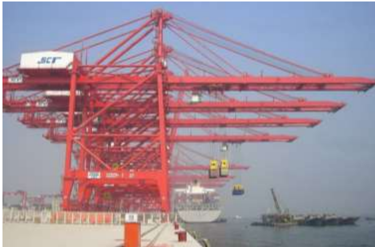
Figure 1. Tandem hoist system.
