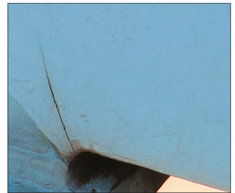
Photograph 2: A typical crack in a fracture critical member on a container crane. This crack can be repaired.
