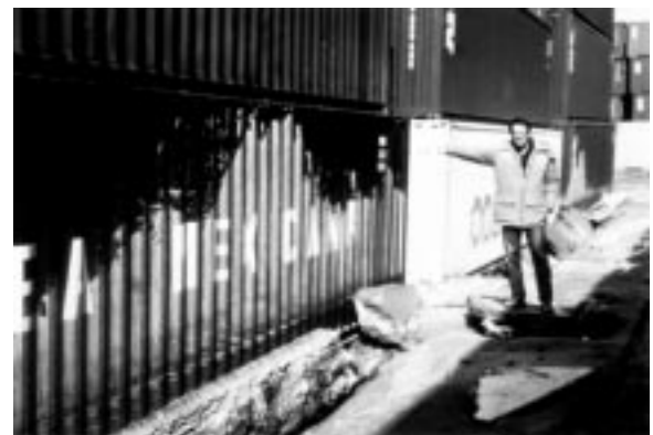
LIQUEFACTION SIGNATURE
