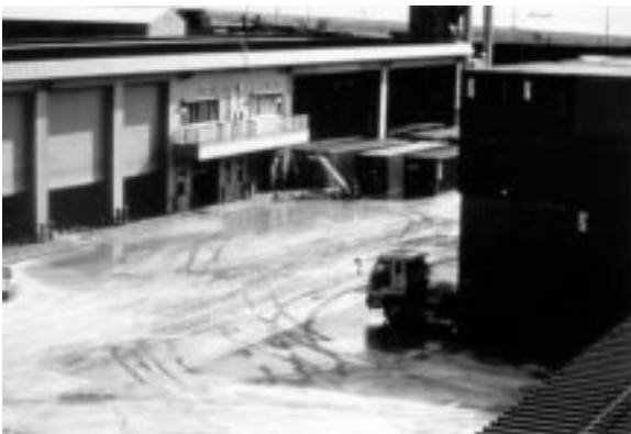
SOIL FINES CARRIED TO THE SURFACE
