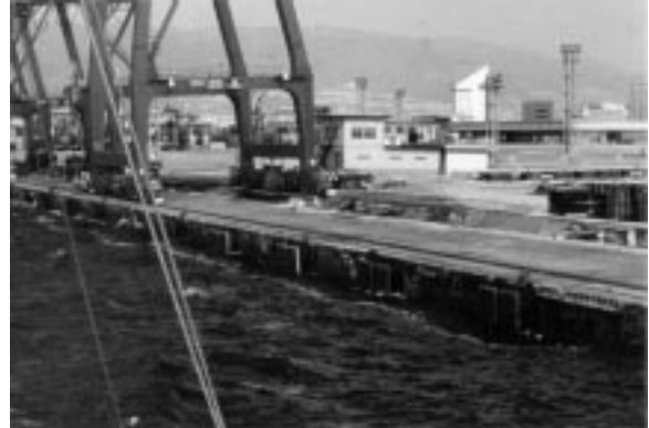
DUCTILE FRAMES PERFORMED WELL
