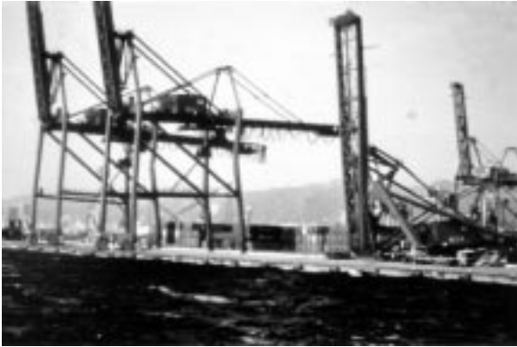
CRANE DAMAGE
