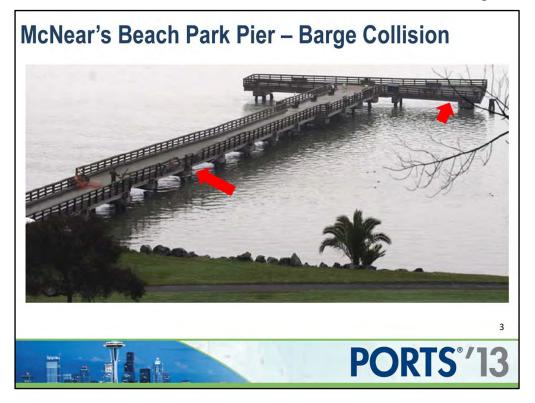
In 2008, a barge broke its mooring during a storm and collided with the McNear's Beach Park Pier, resulting in significant damage to approximately half of the structure.
