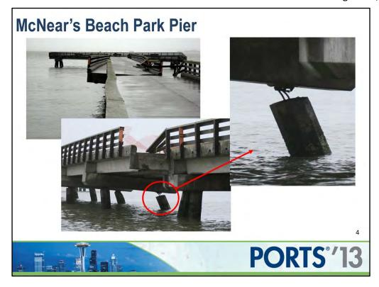
These photos show the end of one pier section displaced 5' laterally after the accident, the resulting pile damage, and the modest reinforcing in the pile connection.
