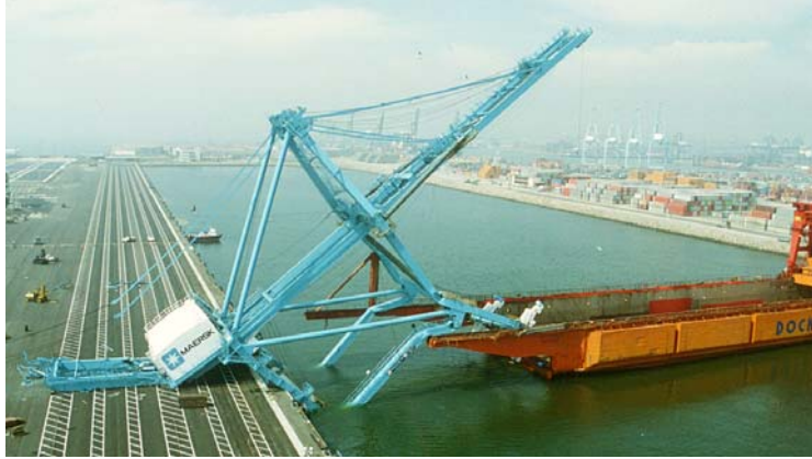
Figure 7. Crane collapse during offloading
