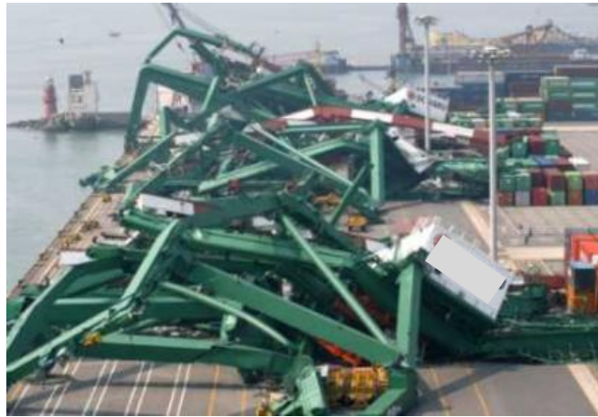
Figure 4. Six cranes collapsed cranes on wharf after typhoon
