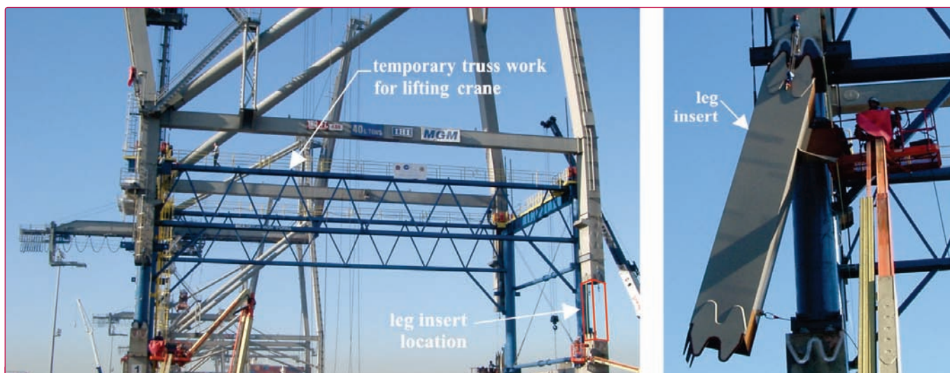
Figure 1. Leg insert crane raise method.
