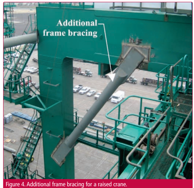
Figure 4. Additional frame bracing for a raised crane.
