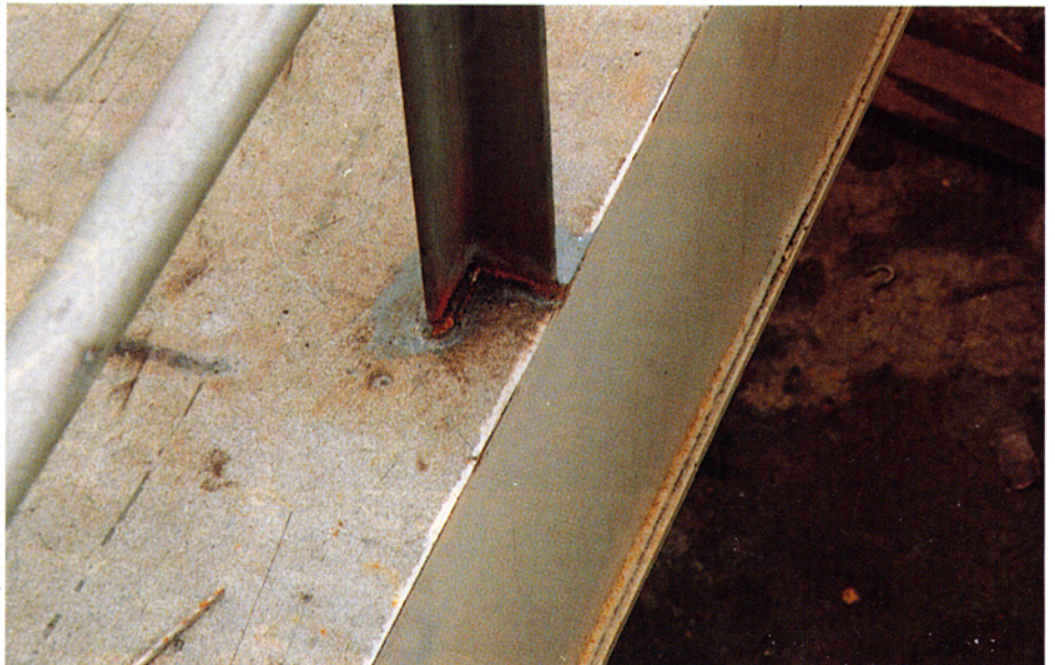
Repaired pipe diagonal
