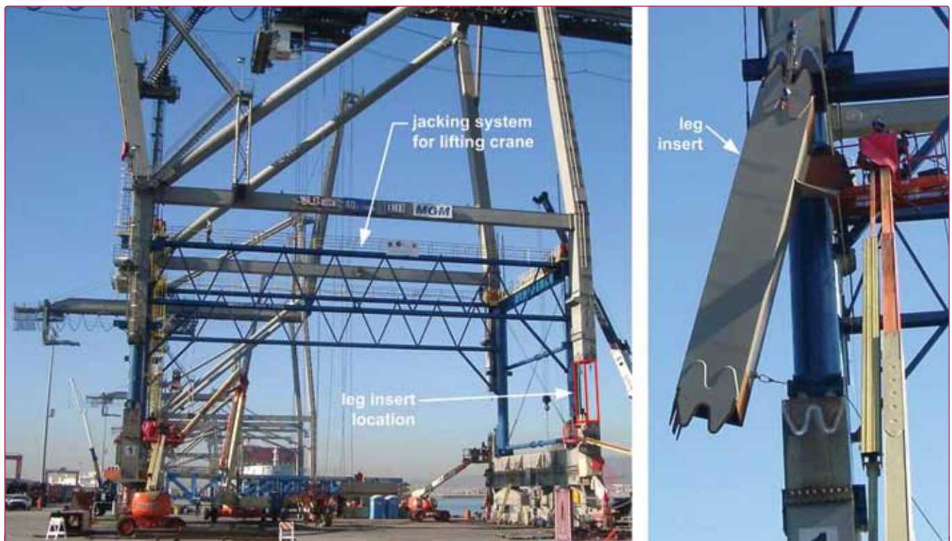
Figure 4. Crane raise and leg insert installation.
