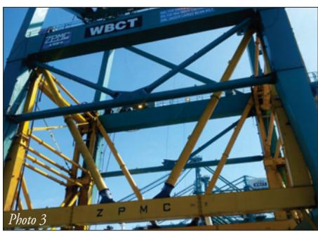
Photo 3: The raised cranes with the new section installed
