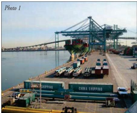
Photo 1: Crane components for several cranes at the site before the start of a crane rise
