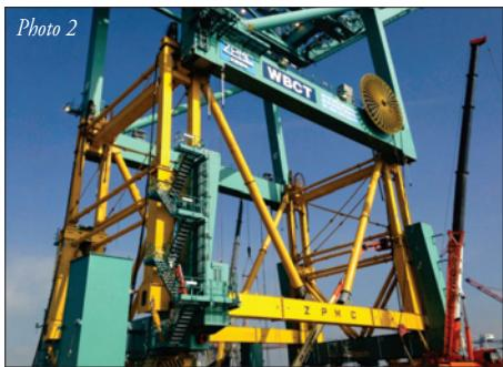
Photo 2: Raised crane on jacking frame, with the new leg sections on the ground
