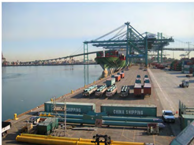
Photograph 1: Crane components for several cranes at the site before the start of a crane raise
