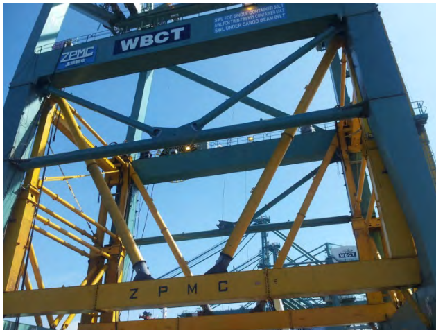
Photograph 3: The raised cranes with the new section installed
