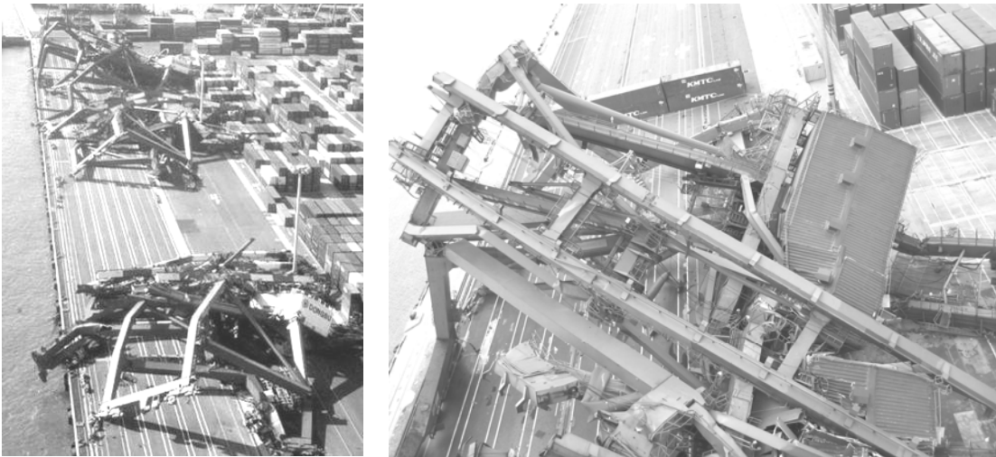
Figure 2. Dockside crane collapses in Korea caused by Typhoon Maemi, 2003
