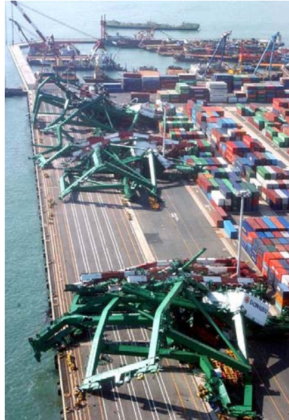
Figure 3: Collapsed Pusan Cranes
