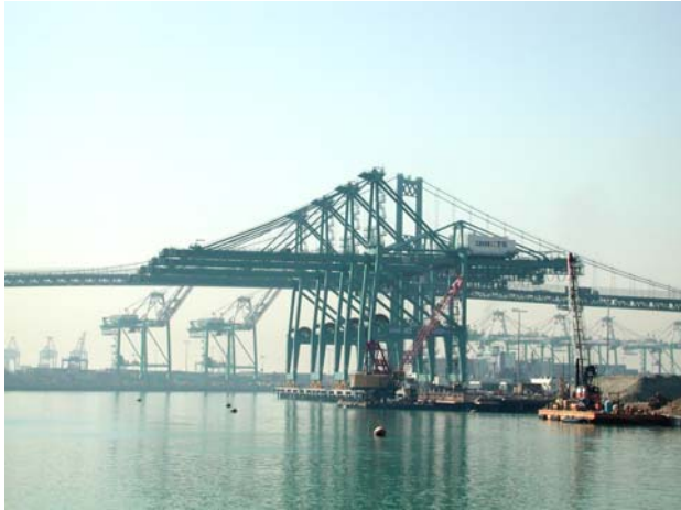
Figure 10: Existing Cranes at the China Shipping Terminal, POLA
