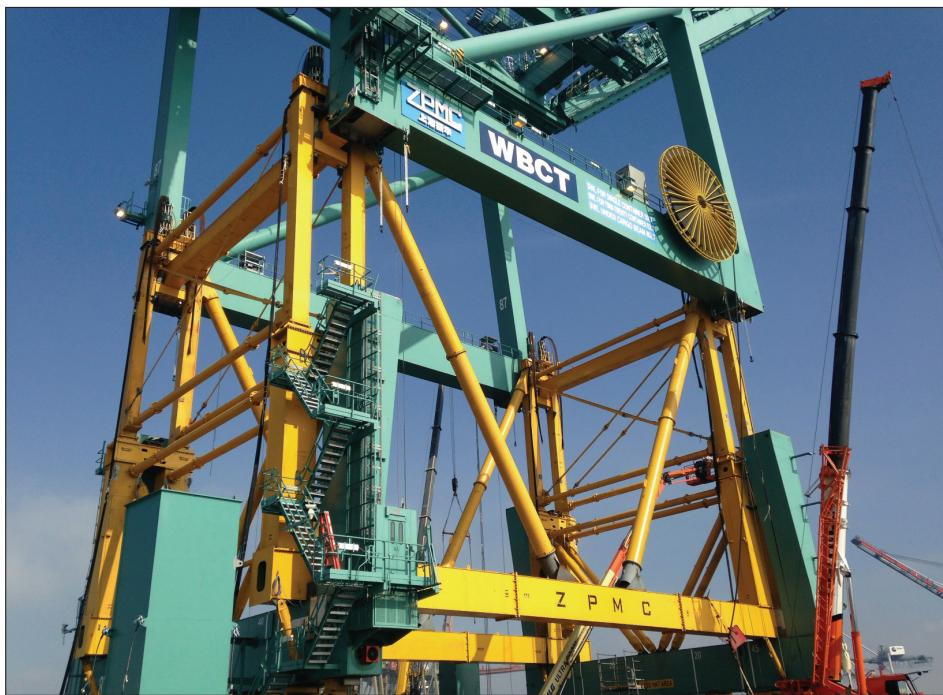
Figure 3: Crane being raised with a jacking frame
