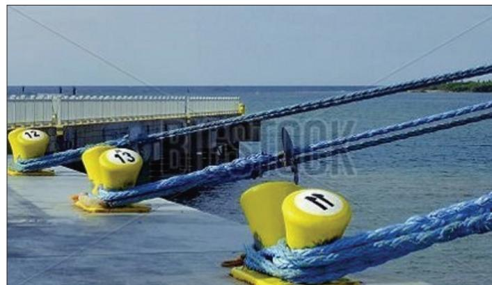
Figure 5: Suboptimal mooring line arrangements - all lines on one bitt
