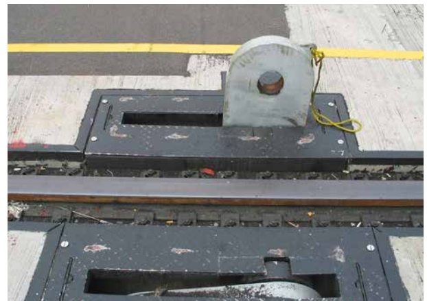
Photograph H: STS crane rail and twin tie-down hardware in a different configuration
