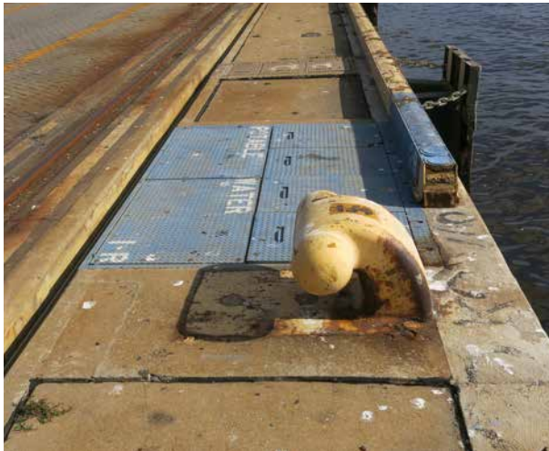
Photograph P: STS crane open waterside cable trench
