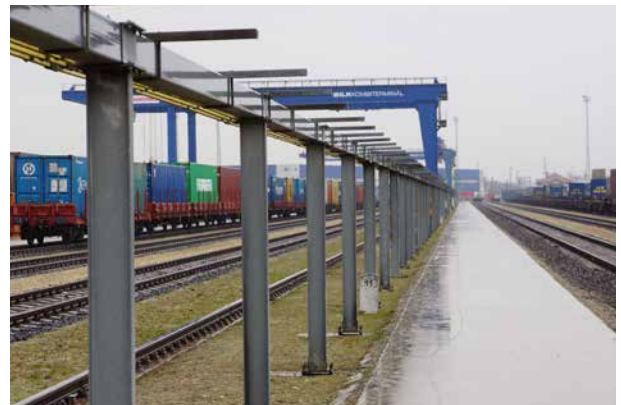
Photograph R: RMG crane with elevated bus bar power supply
