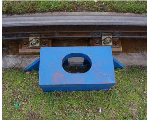
Photograph E: RMG crane pin socket
