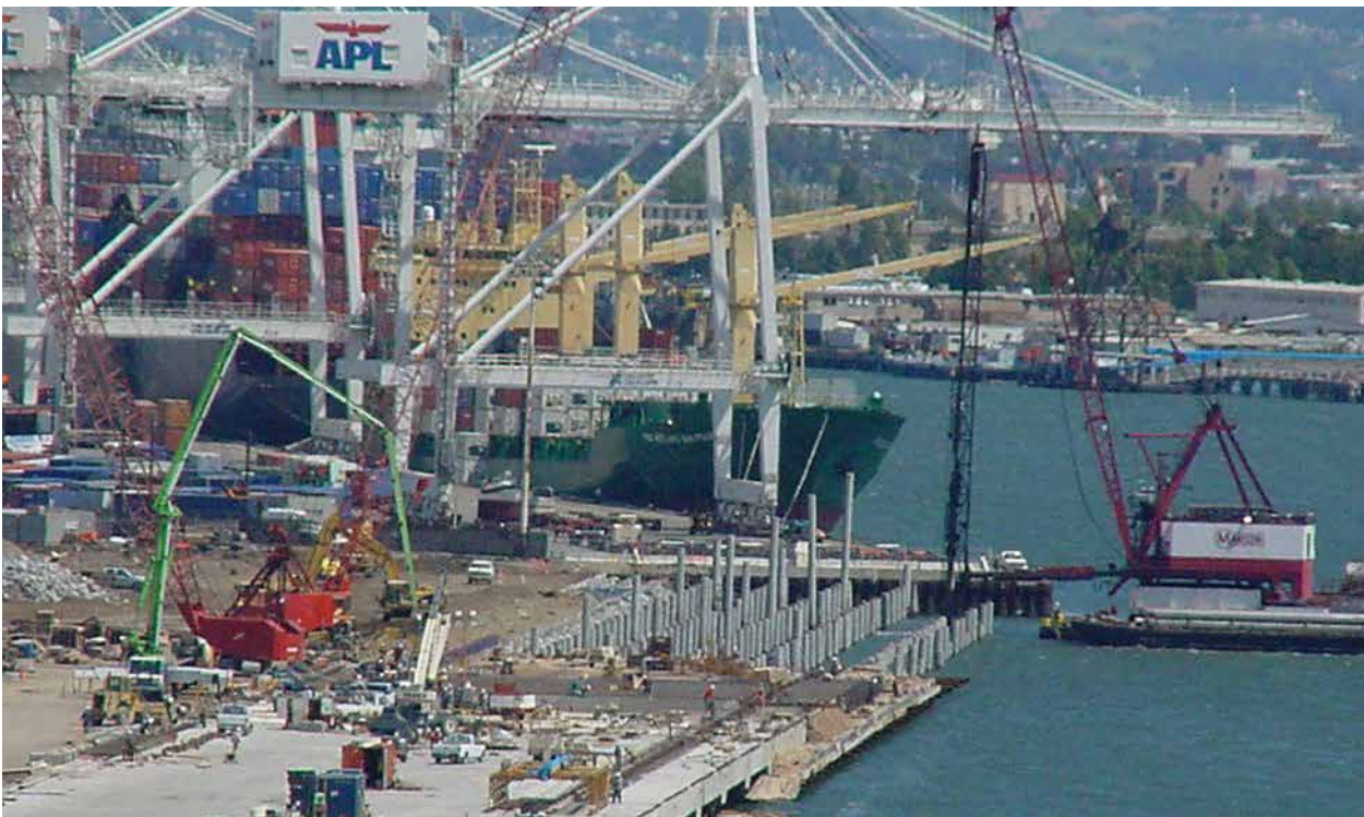
Photograph C: Construction of STS container crane wharf
