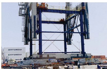
Top: Figure 4. Mooring dolphin at IMTT Port of Richmond; Bottom: Figure 3. Crane being raised with a jacking frame
