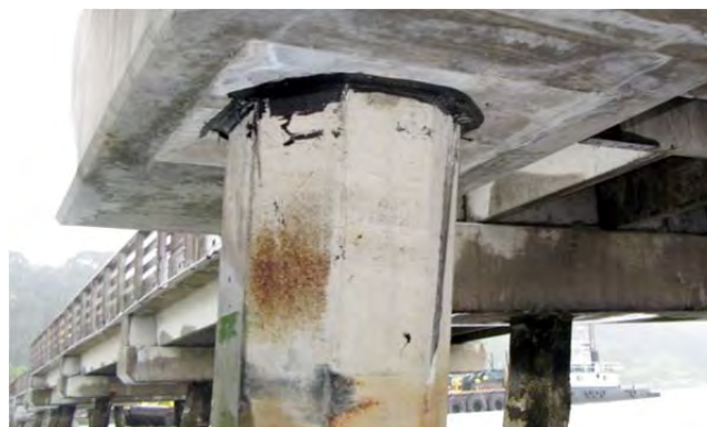
Figure 6. Photograph of sealed pile connection.
