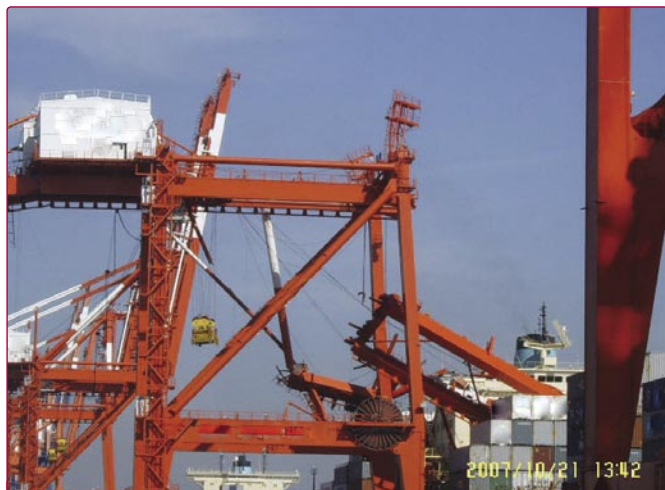
Figure 1. Crane boom failure. Asia – October 2007.
