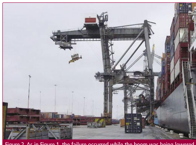
Figure 2. As in Figure 1, the failure occurred while the boom was being lowered. Europe – January 2008.
