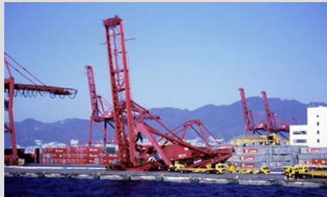
Kobe - Liquefaction
