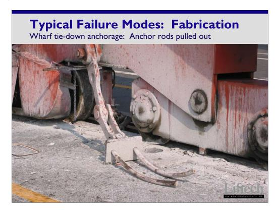
This photo shows the anchor rods pulled out of the wharf.
