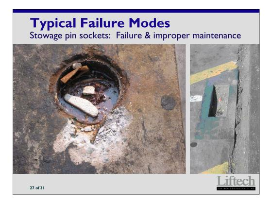
The stowage pin sockets are sometimes filled with debris. Photo on left shows a failure whereby the tie-down had already failed, but the amount of uplift required to lift out of the hole appears minimal.
