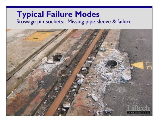
Socket on the left has no reinforcement pipe. This results in transfer of the entire load to the other pin.
